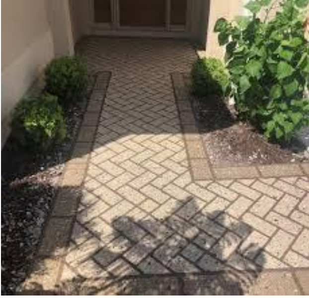
Image # 4 Brick paver walkway leading to screened-in porch
