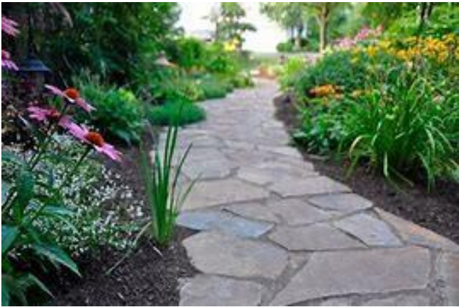
Photo # 9 Irregular flagstone walkway leading from back yard patio to pool
